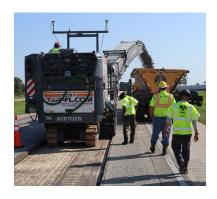
The combination of top-flight equipment — TIP's Wirtgen W210 Fi features a 7'-wide mill — and the RD-MC solution, helped Ajax achieve production rates of up to 3,000 ft./day. According to Hunt, using the enhanced milling approach also streamlined the paving effort, which followed on the heels of the milling.
