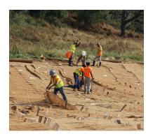
In the case of accurately placing larger boulders, which generally weigh 3-4 tons, Bourn's excavators dig deep into the stream's subbase so the top of the structure can hold grade and create a pool after it, according to Steve Griffin, Bourn's foreman.
