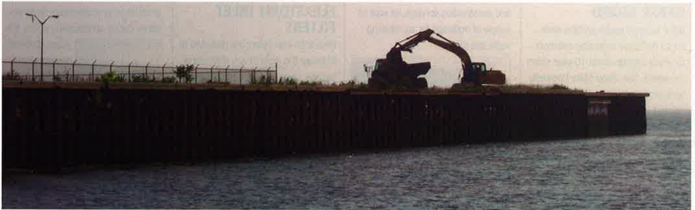
The shoreline at the Floyd Bennett Field Marine Corps Reserve Center in Brooklyn, NY, recently required stabilization. A deteriorating steel wall (above) was replaced with a stone revetment wall (below).
