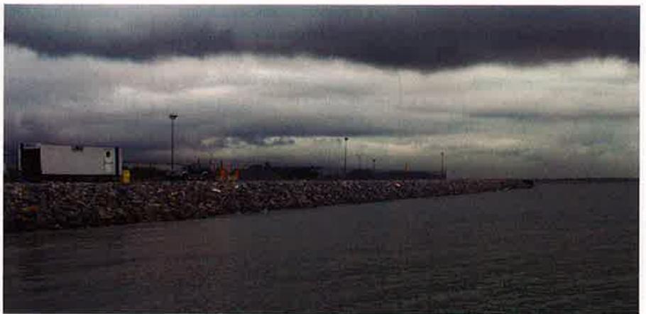
The shoreline at the Floyd Bennett Field Marine Corps Reserve Center in Brooklyn, NY, recently required stabilization. A deteriorating steel wall (above) was replaced with a stone revetment wall (below).
